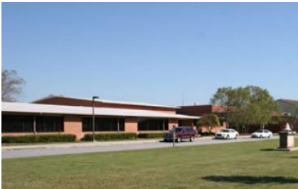
Phase 1: EnergyCenter HVAC controls were installed at Franklin High School.
